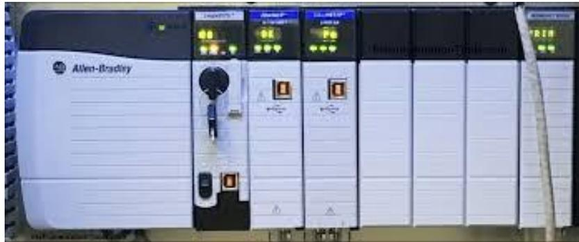
Figura 53 PLC Allen Bradley 1756 -PA75/A
