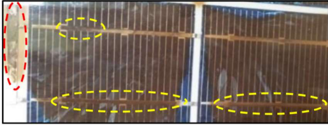
Figure 1.1: Corrosion in PV panel. Adapted from: [6]
