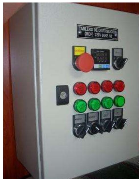
**Figura 12.** Tablero de control para Chiller (COPELAND, 2009)
